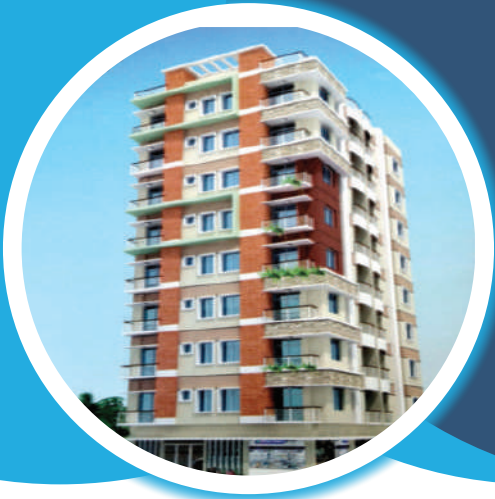
Project: A One Housing & Development 02 Client Name: Md. Swiod Shhainuzzaman Description: (9th Storied) 2400 Sft Bashundhara, Block-B, Baipail, Ashulia, Savar, Dhaka
