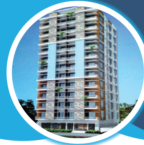
Project: A One Housing & Development 01 Client Name: Md. Swiod Shhainuzzaman Description: (12th Storied) 2400 Sft Bashundhara, Block-B, Baipail, Ashulia, Savar, Dhaka
