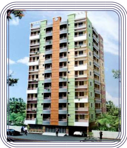
Project: Mother Tower Client Name: Md. Shajahan Ali Description: (15th Storied) 1500 Sft Namira Village, Bashundhara, Block-A, Baipail, Ashulia, Savar, Dhaka
