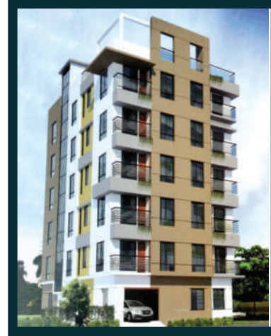
Project: Mafuz Tower Client Name: Md. Anwerul Haque Mahfuz Description: (6th Storied) 3000 Sft Bashundhara, Block-A, Baipail, Ashulia, Savar, Dhaka
