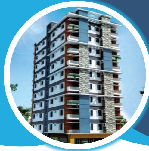
Project: A One Housing & Development 03 Client Name: Md. Swiod Shhainuzzaman Description: (10th Storied) 2600 Sft Bashundhara, Block-B, Baipail, Ashulia, Savar, Dhaka
