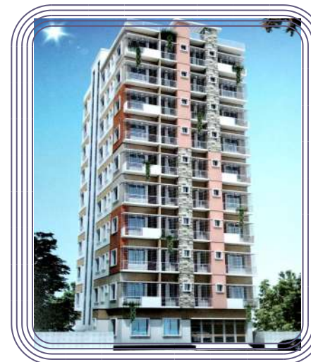
Project: Sara Tower Client Name: Md. Elias Hossain Gong Description: (10th Storied) 3000 Sft Bashundhara, Block-A, Baipail, Ashulia, Savar, Dhaka
