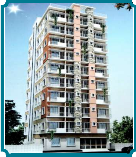
Project: Bashudhara Sky Line Client Name: Md Atik Hossain Gong Description: (10th Storied) 3000 Sft Bashundhara,Block-A Baipail, Ashulia, Savar, Dhaka
